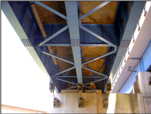
橋梁補修施工前
