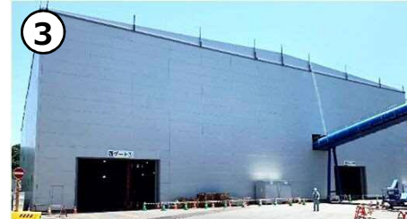
③-1 発進立坑地上設備(R1.6時点)
