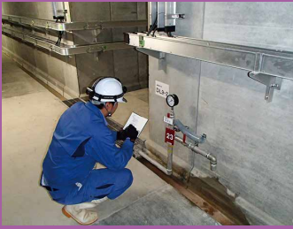
Dam body inspection
