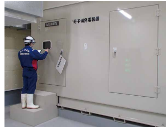
Telecommunication equipment inspection
