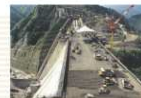
Construction of the RCD concrete method (1983)
