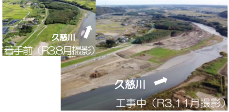
②R2久慈川左岸富岡地先築堤護岸外工事
