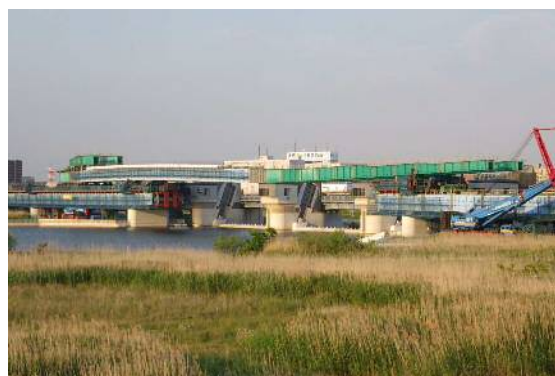
送出し架設施工状況
