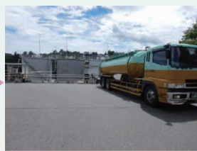
Limestone is stored in large silos at the Neutralization Plant
