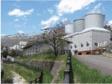
Neutralization Plant of Kusatsu
