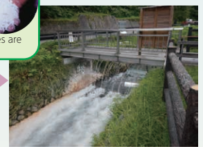
The resulting limewater is returned to the river to neutralize it
