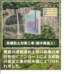
In Tochigi Prefecture, work to fix the bedrock using anchor works to prevent the progress of the collapse of the upper part of Kegon Falls Waterfall Platform was carried out.
