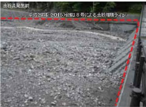
Before the debris flood occurred Debris deposit line caused by Typhoon No. 18 in 2015
