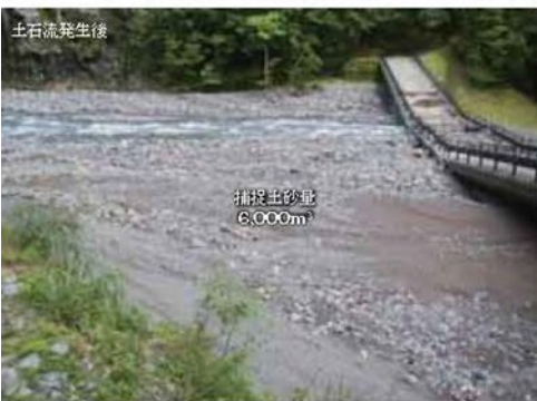
After the debris flood occurred
