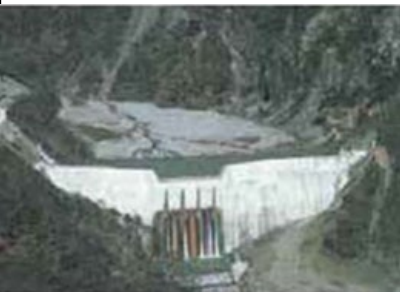
After carrying out the 2nd raising work (1982)
