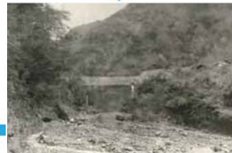
After carrying out the 1st raising work (1953)
