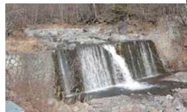
Sabo Dam No. 6
