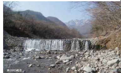
Sabo Dam No. 2
