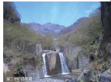
Kamatusawa Sabo Dam
