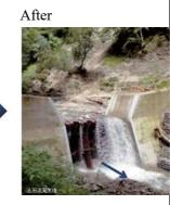
Prevention of damage to 12 houses by trapping soil and driftwood
