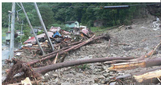
Serizawa District when it was damaged by the Kanto and Tohoku heavy rain disaster in 2015
