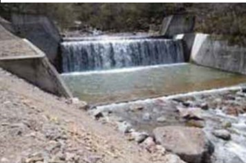
Okukinu Sabo Dam No. 3
