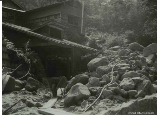
Nikkozawa Onsen (formerly Kuriyama Town) debris flood damage
