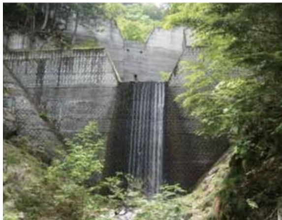
Hacchoyusawa Sabo Dam
