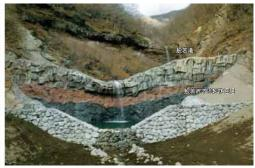
For Hannyazawa Karyu Sabo Dam, a mold was made of the existing rock, an "artificial form" was created, and concrete was poured in. After this, the surface was colored. This cleverly makes it melt into the scenery.
