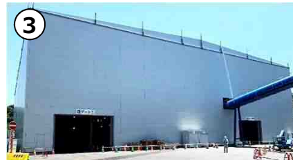
③-1 発進立坑地上設備(R1.6時点)
