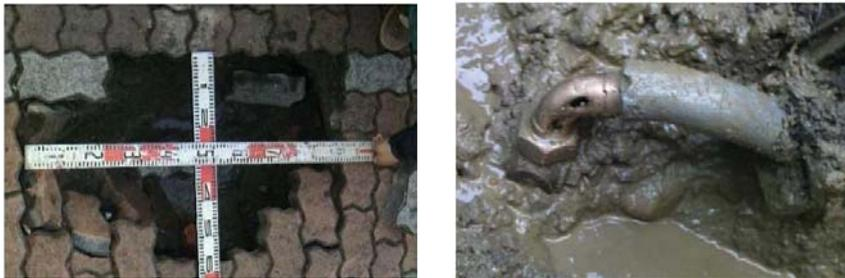
路面陥没 約0.6m×0.9m×0.35m(深さ)
