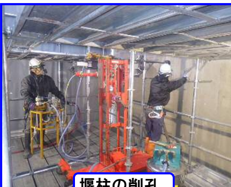
堰柱の削孔
