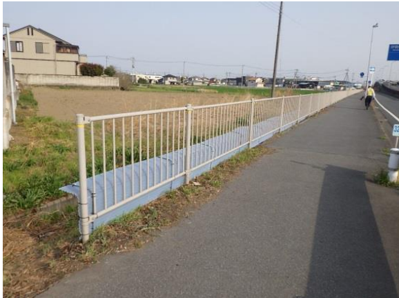
写真-6 つる返し設置状況①
