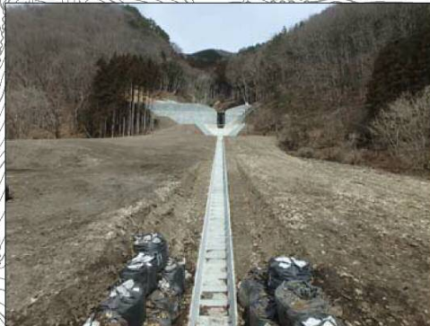
下坪上沢砂防堰堤
