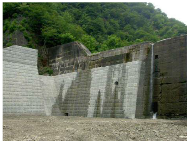
堤体補強施工後
