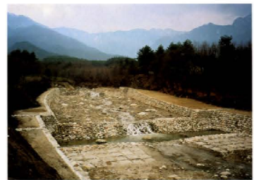
⑪ 大妻川床固群(石室川) Ohmukawa groundfills(Ishitorogawa) 上流には風光明媚な精進ヶ滝があり、河岸にはカワセミも棲む豊かな周辺の環境と調和した施設づくり。 There is a good sightseeing area. Shojigataki waterfall, at the upstream. The facility was constructed with a good balance among the nature where kingfishers reside near the banks.
