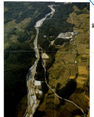
⑦ 尾白川床固群 Ojiragawa groundfills 尾白川合流点から尾白川下流砂防えん堤までの間に下流側を山腹側、上流側を国土交通省が施工した床固群。 This groundfill was constructed between the merge point with Kanagawa river and the Ojiragawa Karyu sabo dam. The lower stream side was done by the Yamana-shi prefecture, and the upper stream side was done by the Ministry of Land, Infrastructure and Transport.
