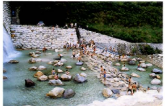
⑥ 尾白川下流砂防えん堤 Ojiragawa Karyu Sabo dam 昭和35年に完成したえん堤に補強、耐震対策を行い、かつ観水水位が高まるよう修繕がなされた砂防えん堤。 The reinforcing work for reinforcement and anti-earthquake feature was performed to the dam completed in 1963. A good accessibility to the river was also concerned during renovation of the sabo dam.
