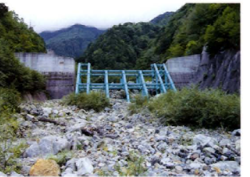
⑬ 大妻川第二砂防えん堤 Ohtanasawa No.2 Sabo dam 関東地方整備局初の鋼製格子砂防えん堤。 This is the first steel-pipe gridded sabo dam in the Kanto Regional Development Bureau.
