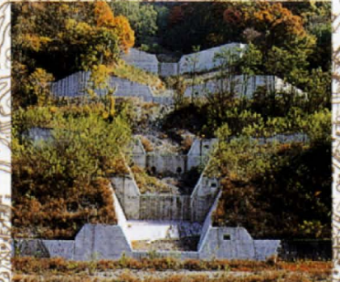
60 釜無山腹工 Kamanashi hillsides works 大原壊れ地を緑にふみかえらせた山腹工 Hillside works which brought back life to the damaged land
