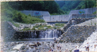
25 武智川上流砂防えん堤群 Takahigawa upper reaches dam 憩いの場の創出と親水性を図った砂防施設 Sabo facilities considering environment and creating a relaxation area
