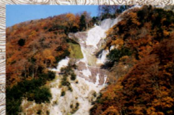
33 釜無本川山腹工 Kamanashi-Honsen hillsides works 釜無川の本川沿いにおける崩壊防止対策施設 Collapse-preventive facilities along the Kamanashi-Honsen
