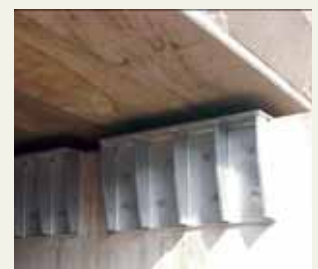
Outer-edge widening brackets to prevent beams from falling off
