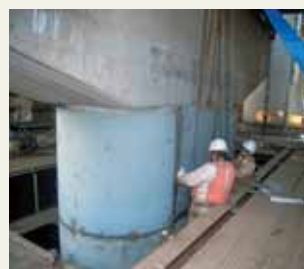
Aseismic reinforcement by winding steel plate around the columns
