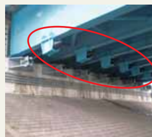
Upper structure (beams) and bottom structure (columns) are connected with cables
