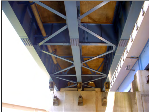
橋梁補修施工前
