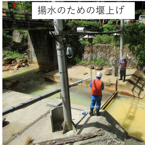
吸水口取付状況 (Suction inlet installation status)
