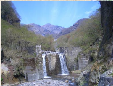
釜ツ沢砂防堰堤
