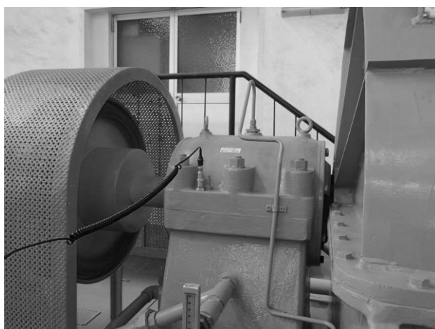
Fig.12 Vibration measurement (fig. 11)
