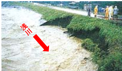
浅川1.2k左岸侵食被害状況(H3)
