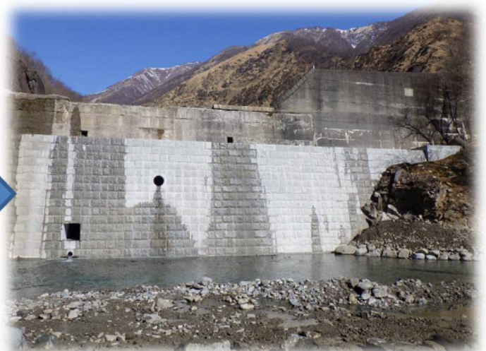
堤体補強施工後
