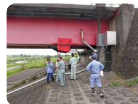
橋梁の履行検査
