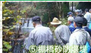
⑤棚橋砂防堰堤
