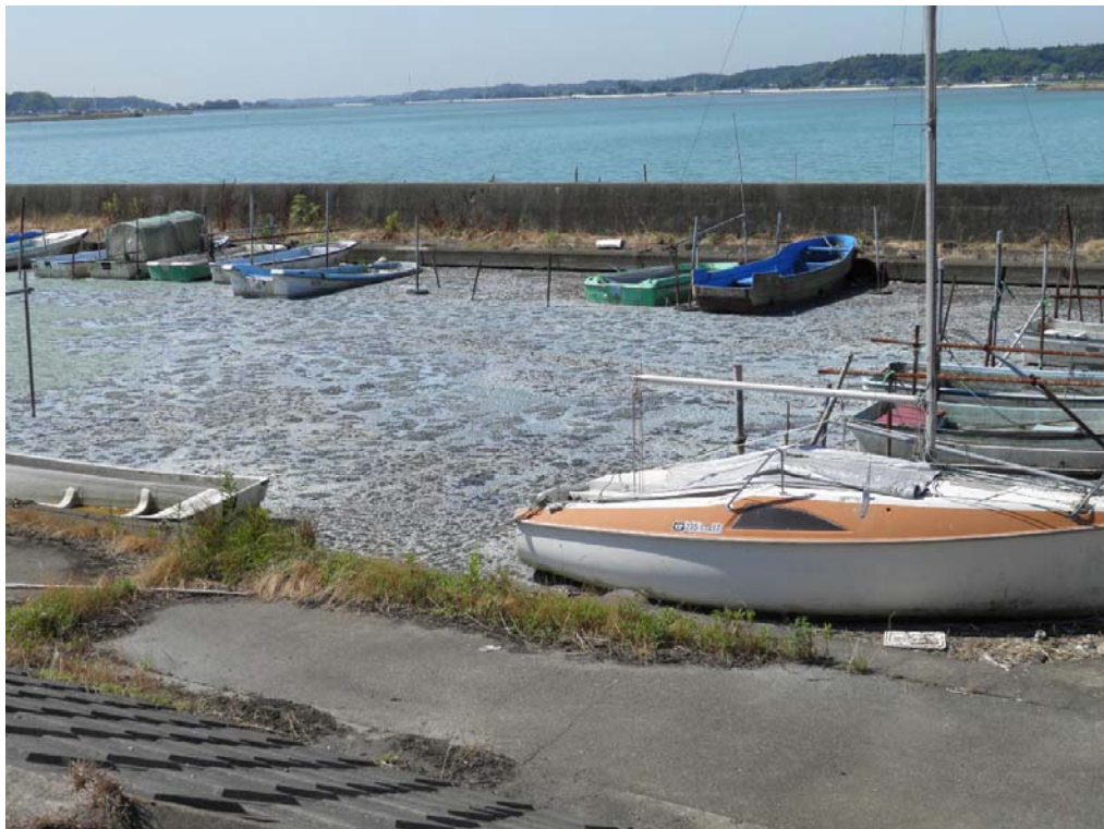
(北浦左岸26.5km+50m安塚舟溜まり内)
